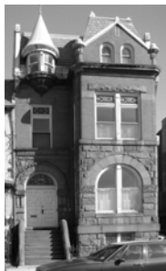
1891 Rabe Residence built [CP]
